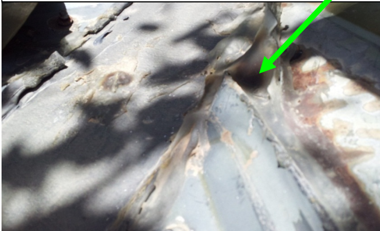
Two panels in different valley areas have split open at the ends of the panels and are temporarily sealed with caulk
